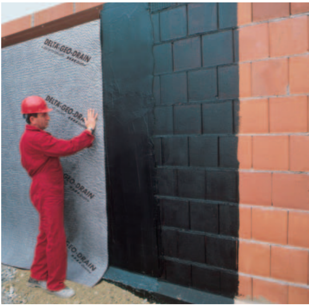
DELTA®-GEO-DRAIN Quattro – a compact unit that can be swiftly installed in one go.
