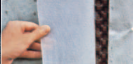
Edge overlap of dimpled sheet and geotextile.
