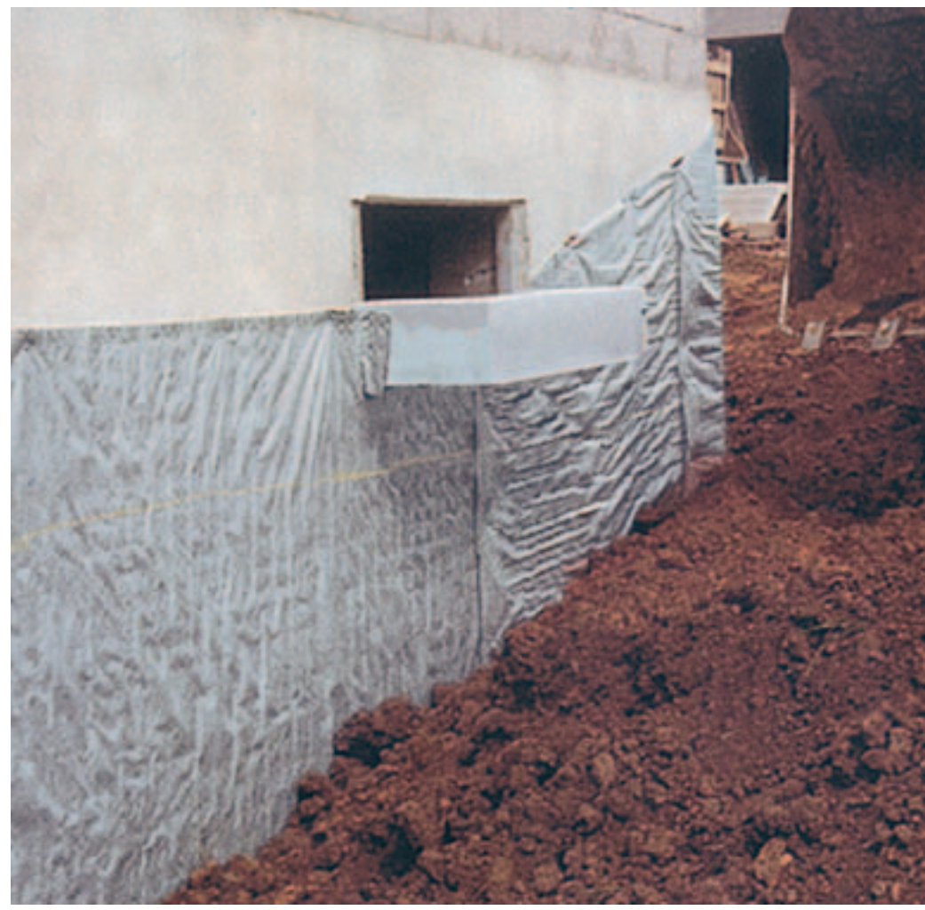
DELTA®-DRAIN keeps foundation walls dry and provides additional heat insulation.
